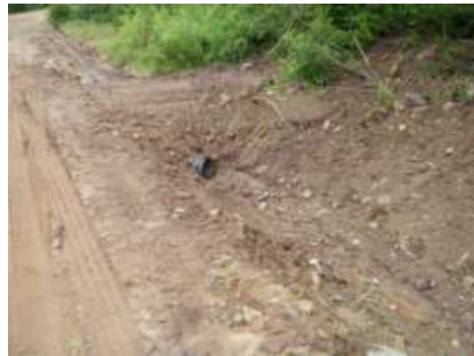
Figure 8 and 9: An undersized culvert on an Irving logging road contributes sediment to a tributary of the Pollett River.
