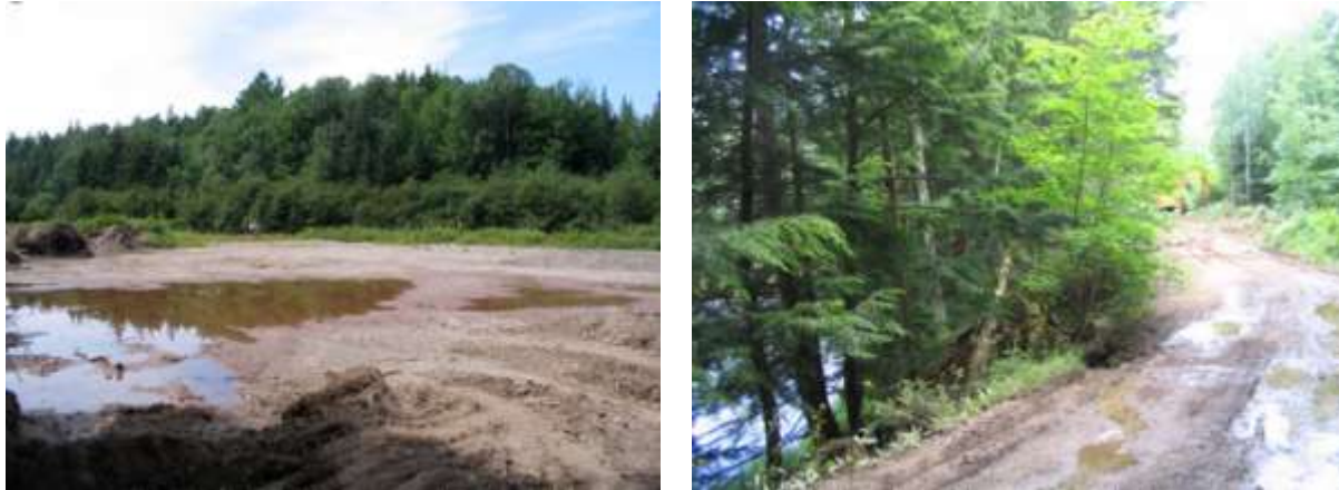
Figure 1 and 2: Damage to Pollett River buffer through removal of gravel (above) and road building activity (above and right) both without the required permits.
