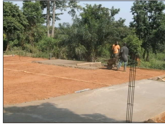
The floor is being put down and soon the walls
